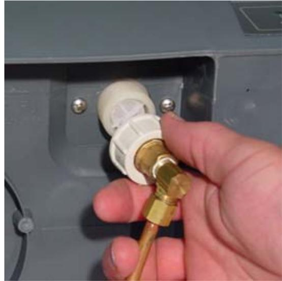
The water feed line should be 1/2" copper, PVC or poly tubing run to within 3 feet of the humidifier, then bushed down to 1/4" O.D. copper or poly to make the final connection to the 1/4" O.D. compression fitting underneath the humidifier. With poly tubing an insert should be used to support the tubing and prevent leaks. This insert is not provided.
