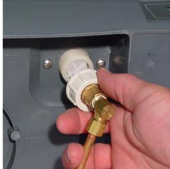
The water feed line should be ½” copper, PVC or poly tubing run to within 3 feet of the humidifier, then bushed down to ¼” O.D. copper or poly to make the final connection to the ¼” O.D. compression fitting underneath the humidifier. With poly tubing an insert should be used to support the tubing and prevent leaks. This insert is not provided.
